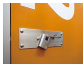
Slide-type locks on individual storage units
