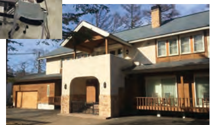
Karuizawa Training Institute & Recreational Facility
