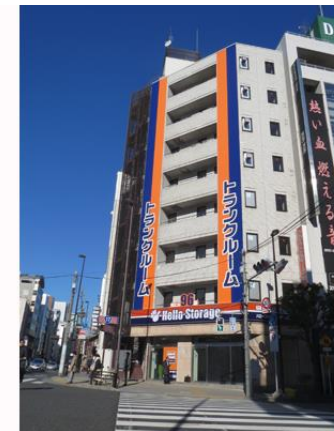
Hello Storage Kanda Akihabara 3(Tokyo)
