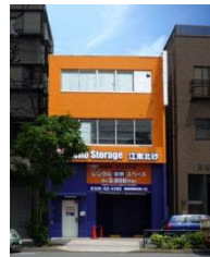
Hello Storage (Room type)
