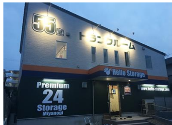
Hello Storage Miyanogi Premier Opened Dec. 2015 (Night view)
