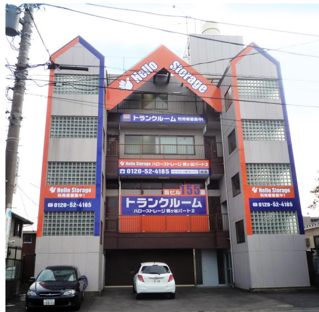
Hello Storage Kajigaya Part 2 (Miyamae-ku, Kawasaki-shi, Kanagawa Pref.) 155 rooms
