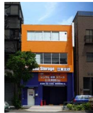
Hello Storage (Room type)
