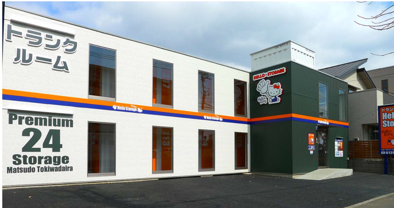
Hello Storage Matsudo Tokiwadaira (system container type) – Opened March 2017
