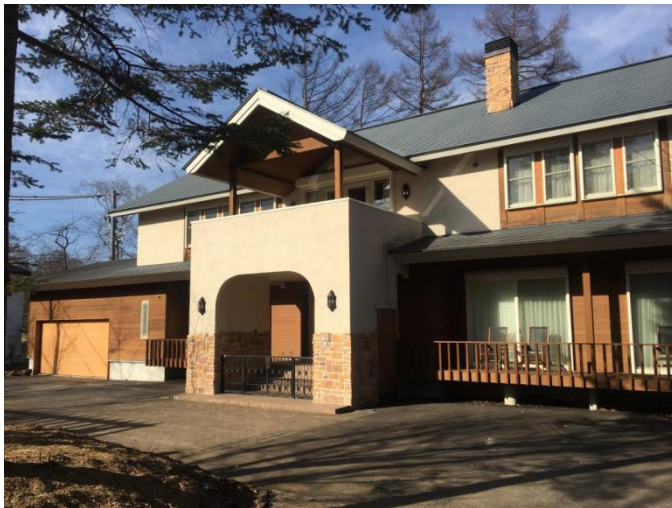
Karuizawa training and recreational facility
