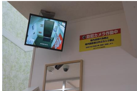
Interior surveillance monitors
