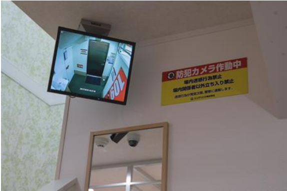
Interior surveillance monitors
