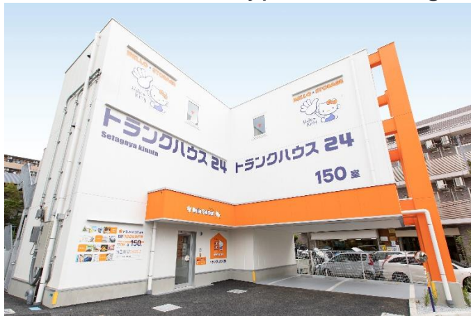
Asset indoor-type self-storage
