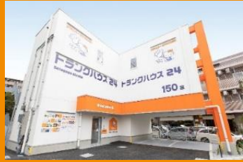
Indoor storage (with land)
