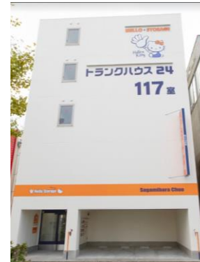
Trunk House 24 Sagamihara Chuo Steel frame structure, 117 units
