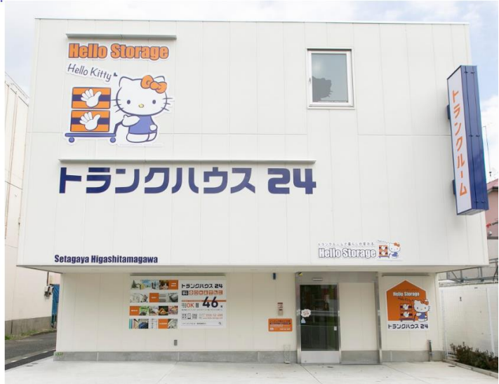
Trunk House 24 Setagaya Higashitamagawa
