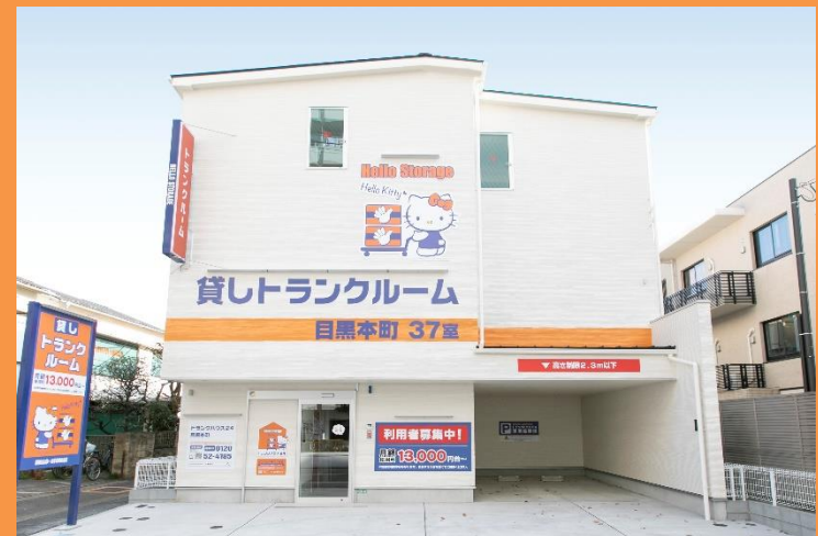
Trunk House 24 (Indoor type) Trunk House 24 Megurohoncho, 38 units
