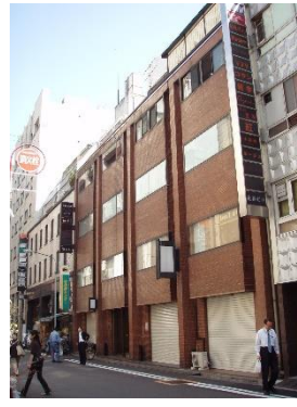
Ginza Idei Building (Chuo Ward, Tokyo)
