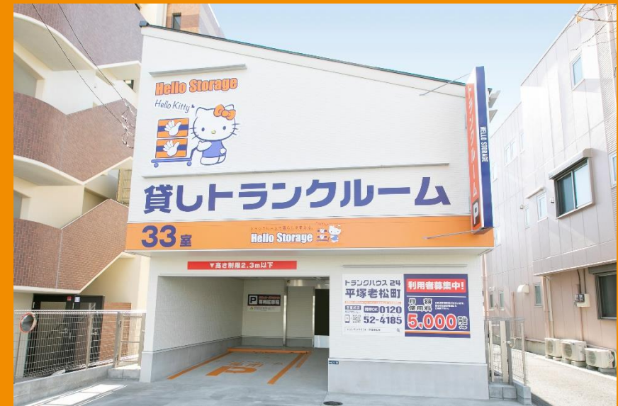
Trunk House 24 Hiratsuka Oimatsucho 33 units
