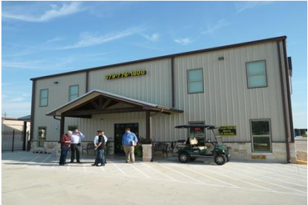
Management office (exterior)
