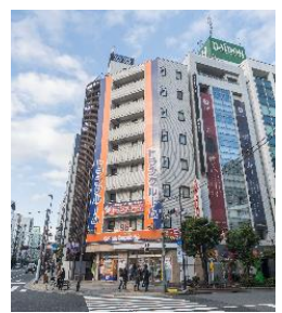
Hello Storage (Room type)
