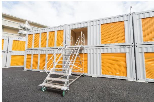
Properties fully equipped with movable staircases
