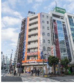
Hello Storage (Room type)
