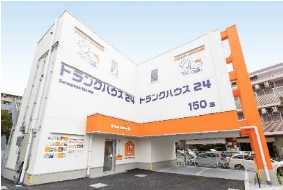
Trunk House 24 Setagaya Kinuta Heavy steel structure, 150 units
