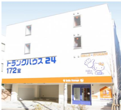
Trunk House 24 Nerima Oizumigakuen Heavy steel structure, 172 units
