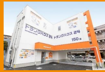
Indoor storage (with land)
