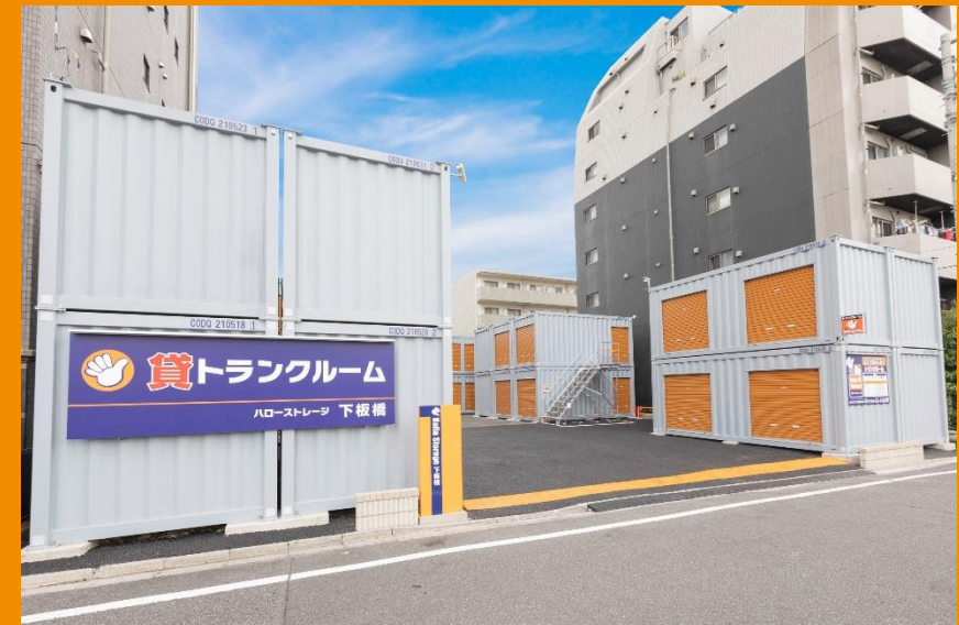
Hello Storage Shimoitabashi, 62 units
