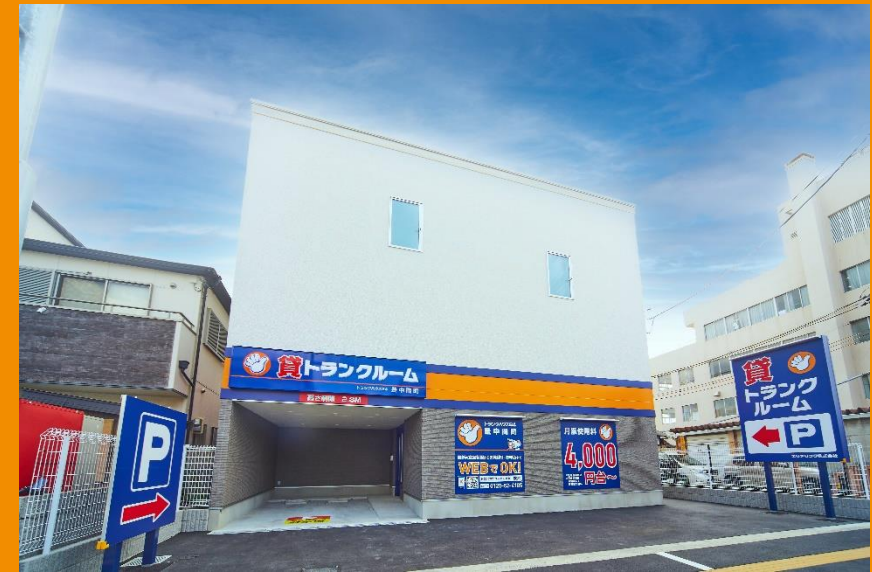
Trunk House 24 Toyonaka Okamachi, 61 units
