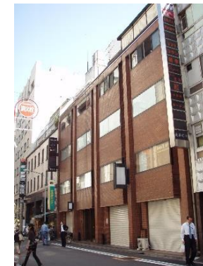
Ginza Idei Building (Chuo Ward, Tokyo)
