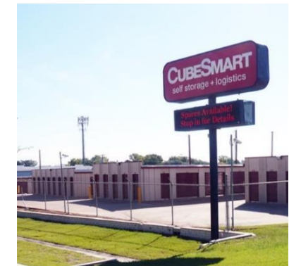
Texas Storage (Texas, U.S.)
