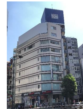
Kanda BM Building (Chiyoda Ward, Tokyo)
