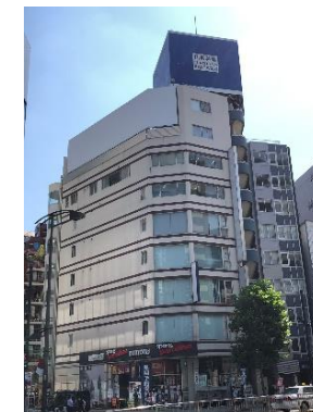
Kanda BM Building (Chiyoda Ward, Tokyo)
