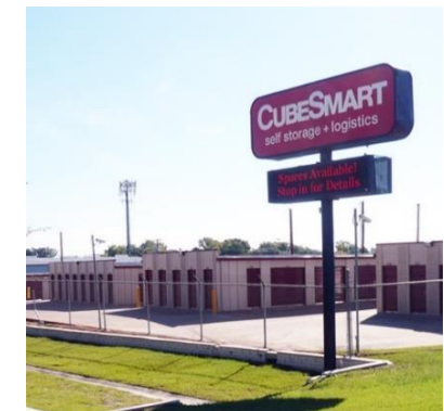
Texas Storage (Texas, U.S.)
